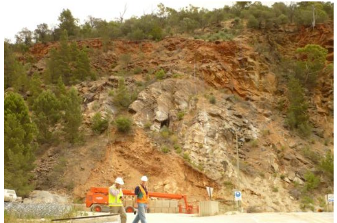
Drilling For The Anchors
