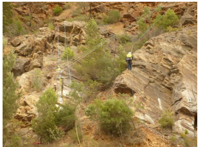
Drilling For The Posts
