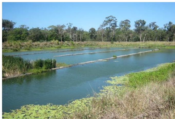
Completed containment pond
