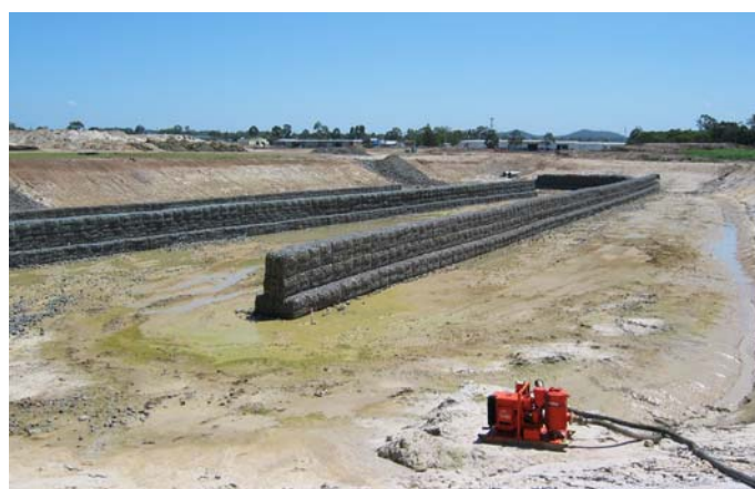
Side perspective of gabion energy dissipator
