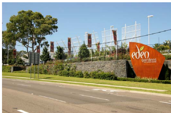
Front view of Gabion wall
