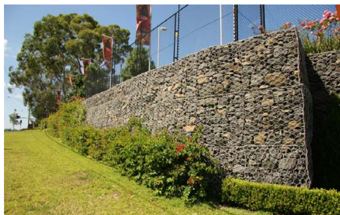
Vertical front face created using gabion formwork
