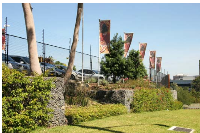
Gabion recess around existing tree
