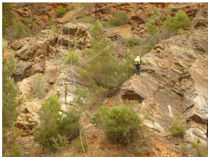
Drilling For The Posts
