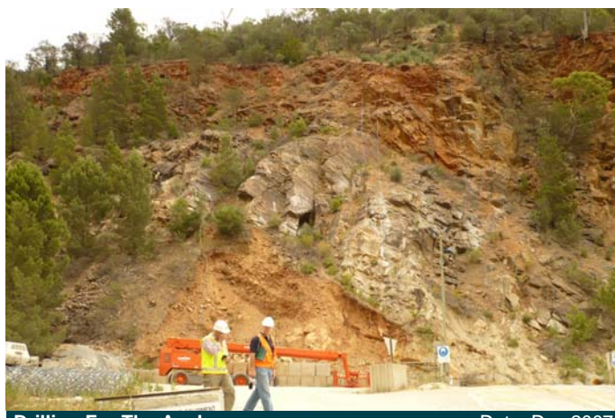
Drilling For The Anchors
