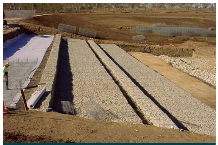
During construction of drop structure
