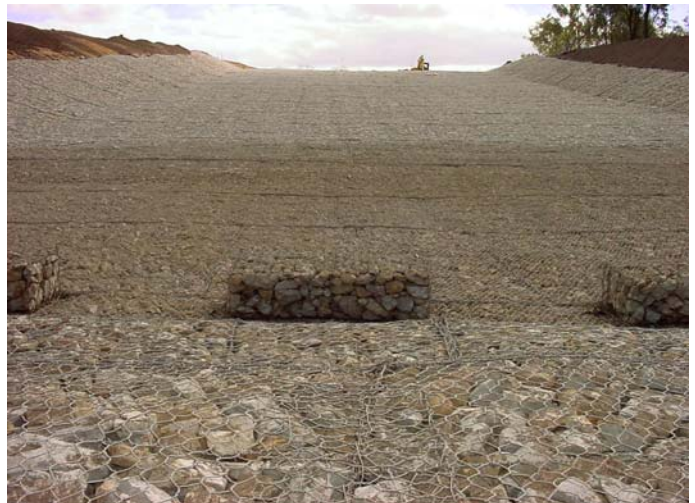
Low wall channel spillway
