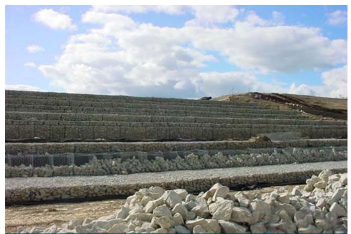
Filling gabion baskets
