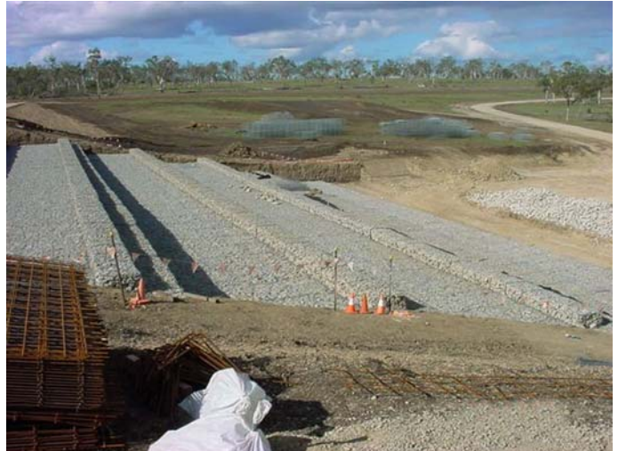
Drop structure almost complete
