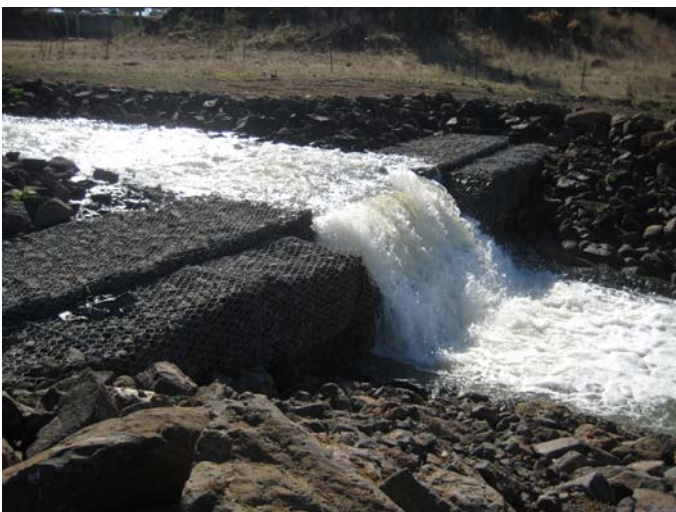
Gabion Drop Structure
