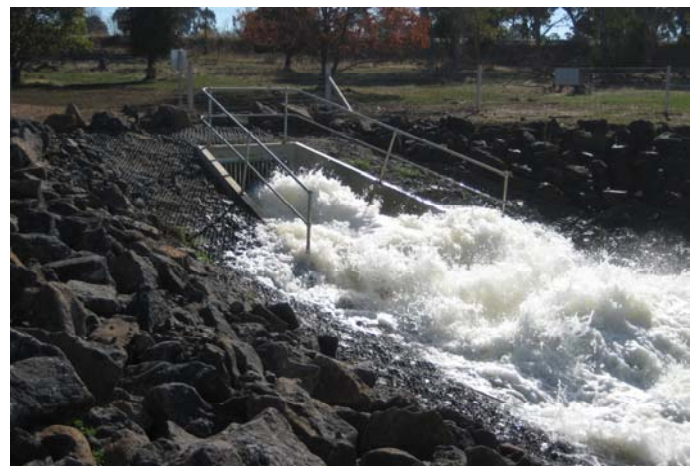
Pipeline Outfall Structure (150ML/Day)
