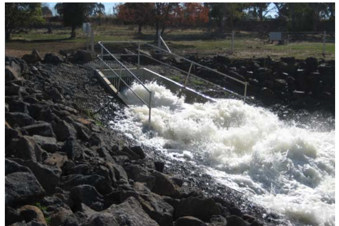
Pipeline Outfall Structure (150ML/Day)
