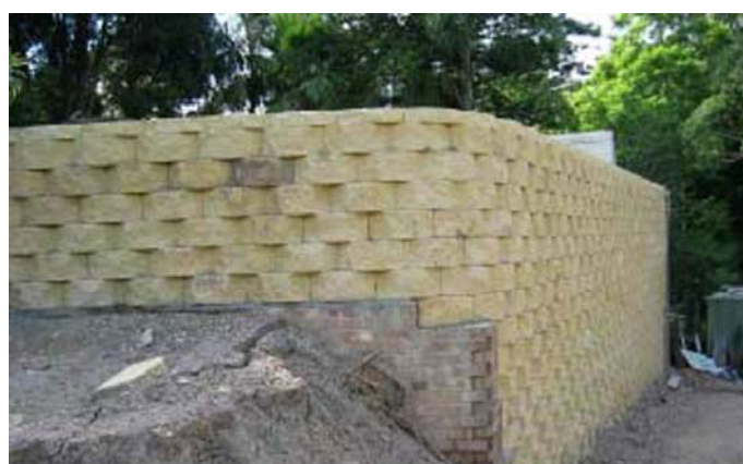
Close-up of segmental block wall
