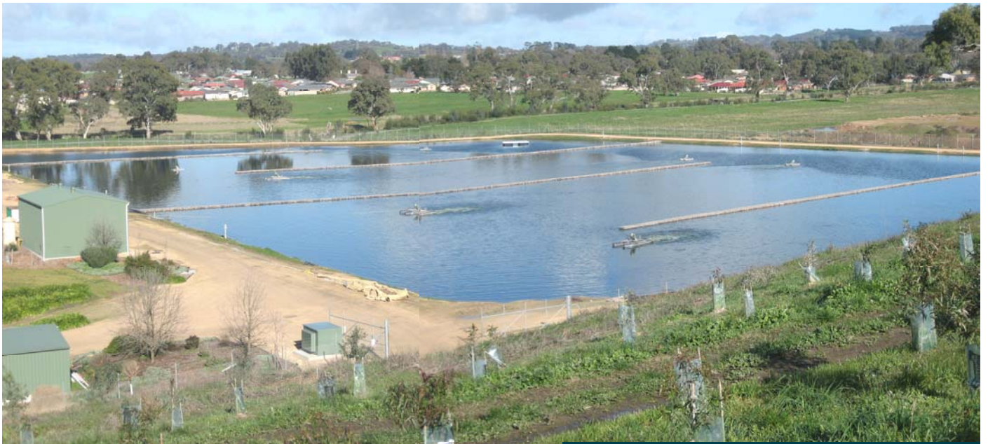
4 Months After Completion
