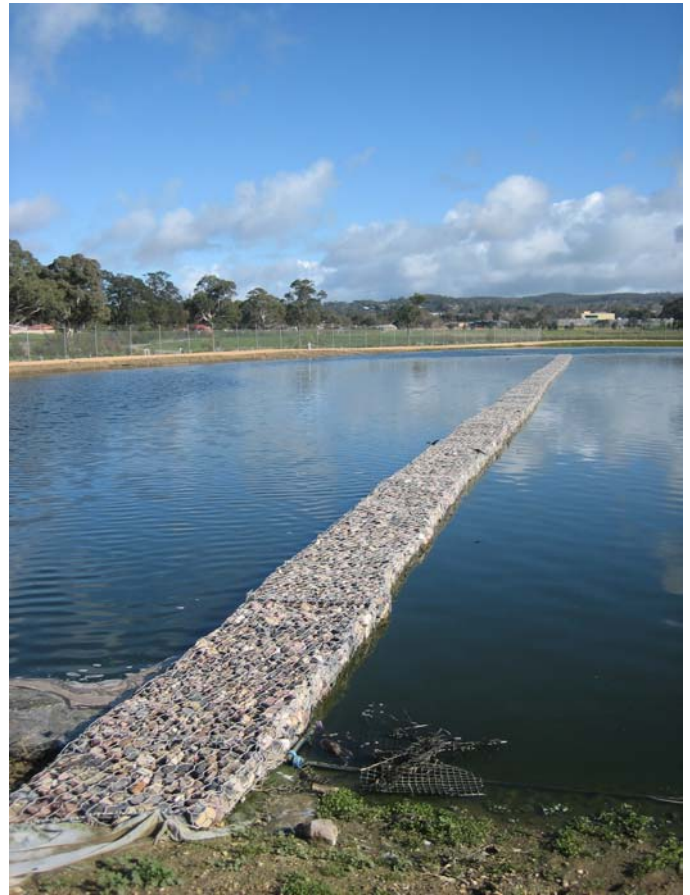
4 Months After Completion
