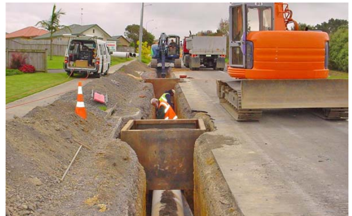
2.3m deep trench with mains pipe
