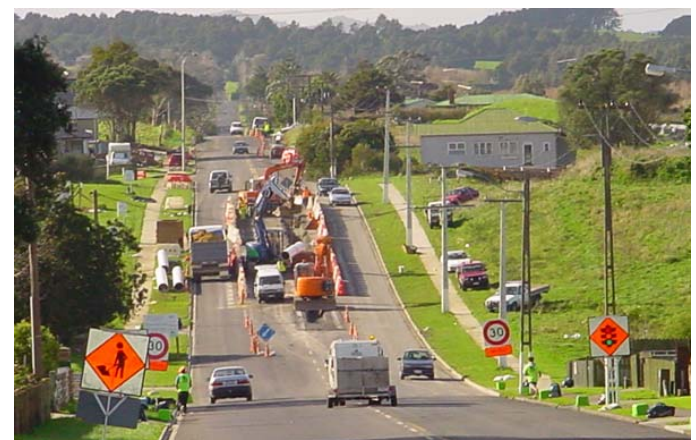
Construction along Alfriston Rd
