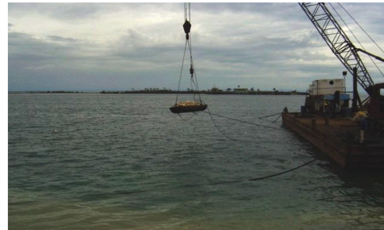
Figure 4. Dumping of secondary armour rock onto seabed.
