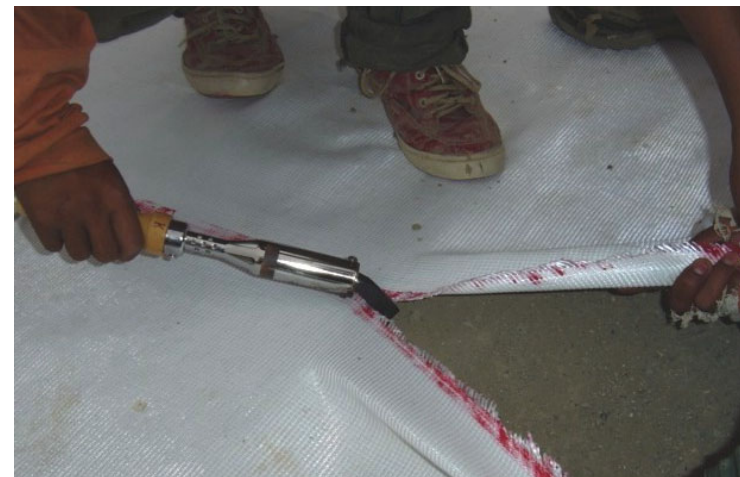
Figure 2. Cutting of geotextile using a heated hot blade.
