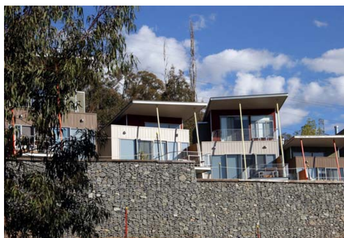
Gabion walls around the Lodges
