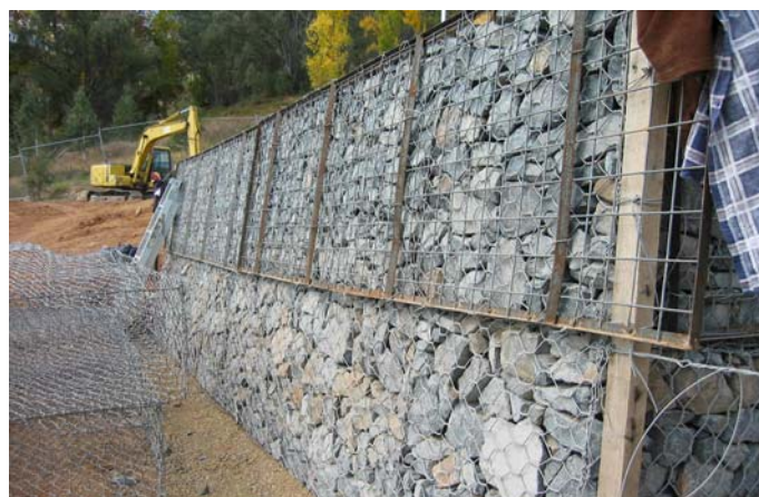
Gabion Formwork to produce straight face
