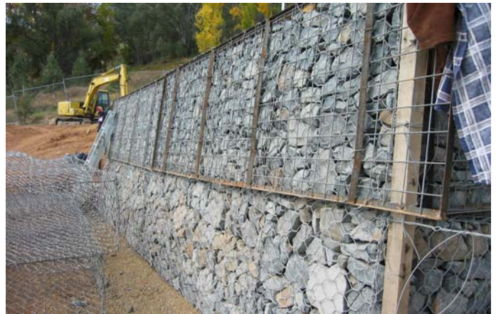
Gabion Formwork to produce straight face
