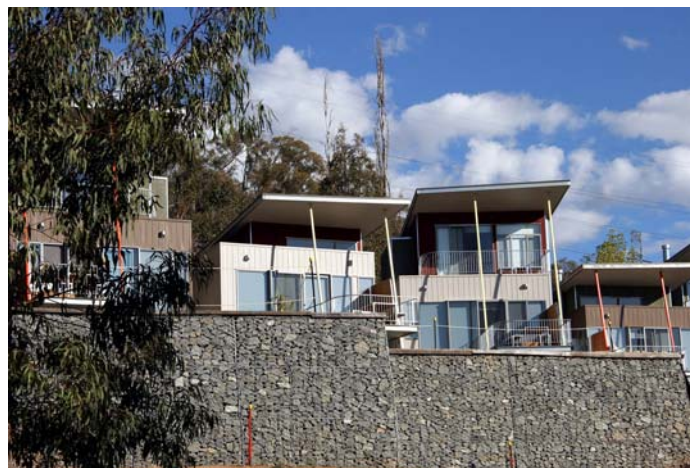
Gabion walls around the Lodges
