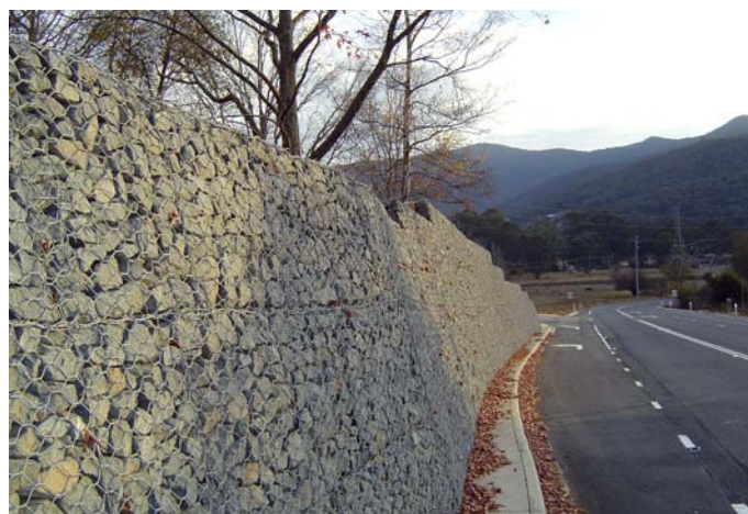
Gabion walls on Bogong High Plains Road
