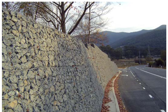
Gabion walls on Bogong High Plains Road
