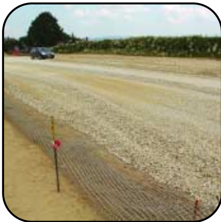
Poland, Żywiec: Sub-base stabilization (Enkagrid MAX)
