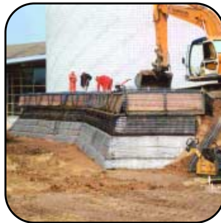
The Netherlands, Emmen: Steep wall using Enkagrid PRO and Enkamat 7210
