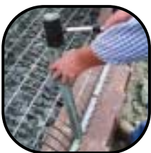
Enkagrid PRO block wall connection detail
