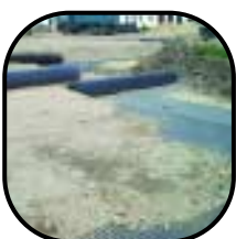
Germany, Altentreptow: Car park
