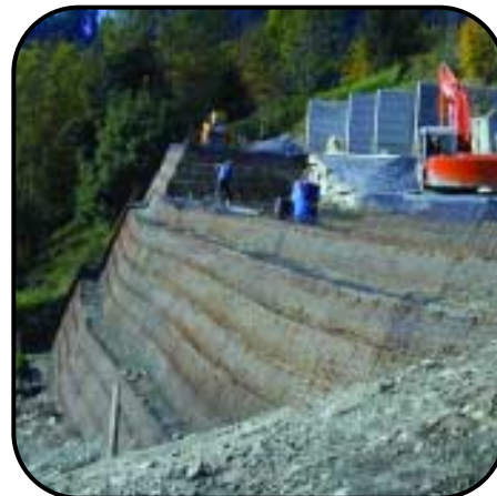
Switzerland, Verbier: Gabion retaining wall reinforced with Enkagrid PRO 40
