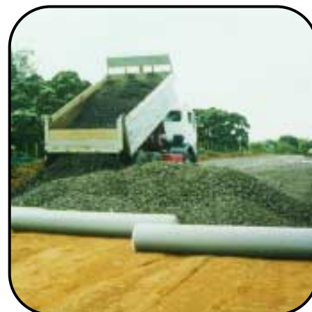
New Zealand, Auckland: Construction haul road using Enkagrid TRC 30
