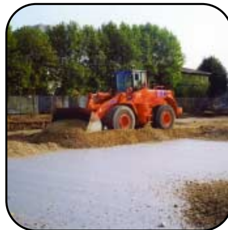
France, Lyon: Soil stabilization construction of a car park (Enkagrid TRC 30)
