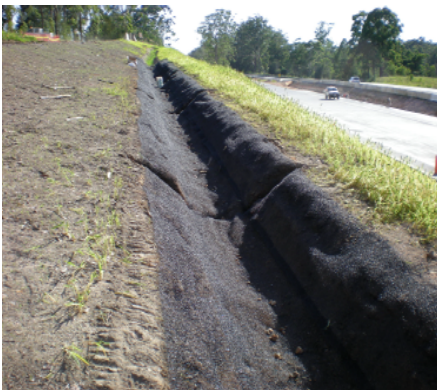
Before: Swale Drain with Enkamat fixed in place
