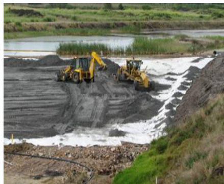
Spreading of fill material over PET layer
