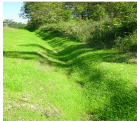
After: Vegetated drain
