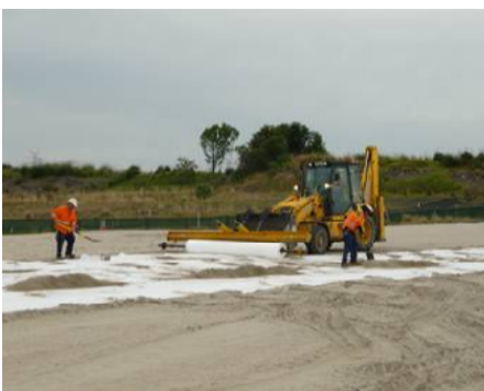
Backhoe with lifting frame laying PET
