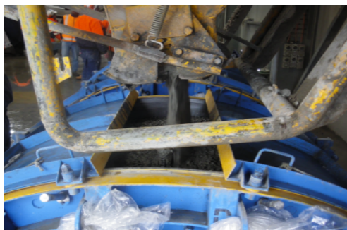
Pouring segment in Bendigo
