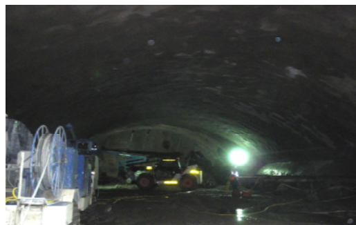
Shotcreting in Adelaide
