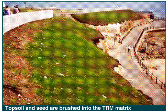
Topsoil and seed are brushed into the TRM matrix
