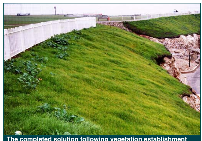
The completed solution following vegetation establishment
