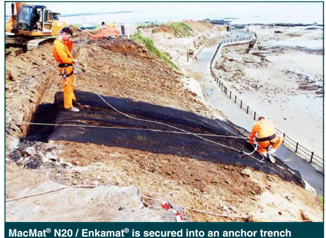
MacMat® N20 / Enkamat® is secured into an anchor trench
