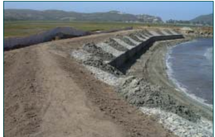
Toppingsoiling of Reno mattresses Date: Oct 2000
